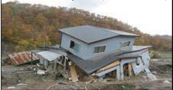
Disaster caused by flood (Hokkaido, 2003)
